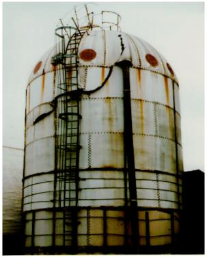
Damage to silo from explosion crack in vapor space
