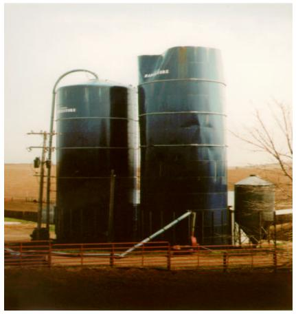
Deformity of silo shell due to explosion
