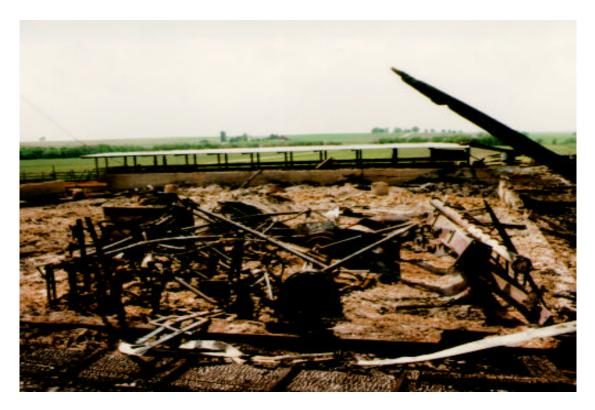
Destruction of farm buildings due to extension of spontaneous combustion - caused fire in silo
