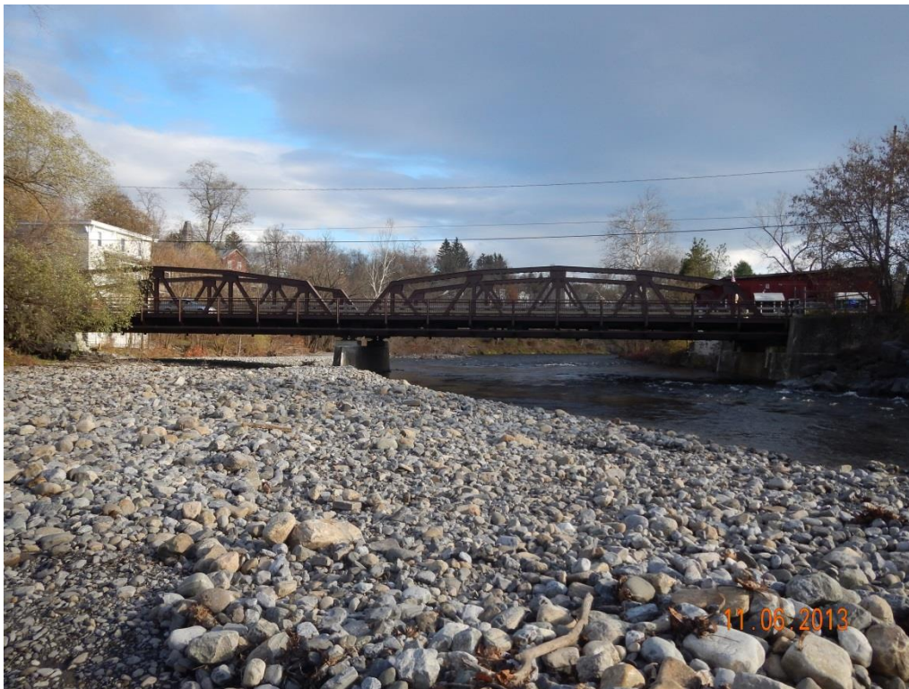
Photo Source: Milone & MacBroom, Inc. (2013)
