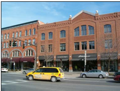
Multi-story, brick façade, build to line.
