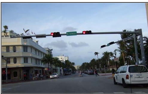
Traffic signal attached to mast arm, no lighting
