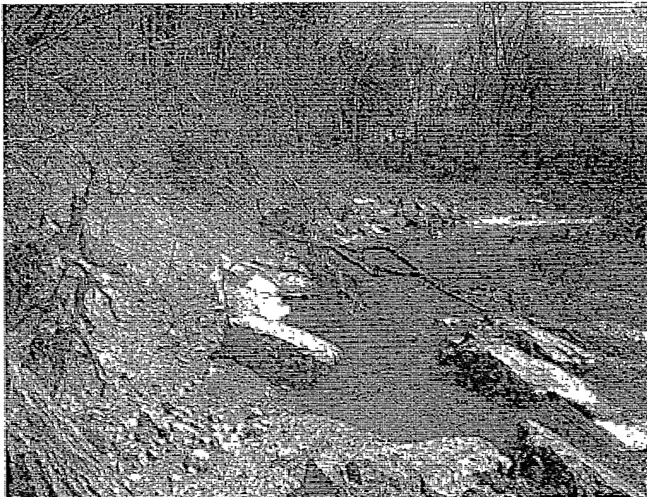
Facing upstream toward erosive east bank on the Sauquoit Creek. The toe of the bank is relatively stable as evidenced by the remaining rip rap. However, in high water events, the flow is erosive enough to damage the upper portion of the banks and undermine the mature trees. The landowner reports losing several trees to the failing bank. Working with the USFWS, we propose that reducing the entrenchment in the Sauquoit Creek will help dissipate flood flows and take pressure off of the upper bank. The cross vane protecting the sewer line is shown upstream.
